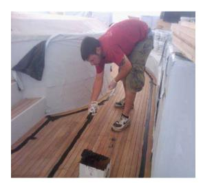
SIS-440 Deck Sealant is a one-part, paste-like neutral cure caulk which, when exposed to moisture in the air, reacts to form a tough, flexible solid rubber compound. The sealant does not sag during cure, and has excellent temperature stability and chemical resistance when cured. Because the sealant is neutral cure, it is non-corrosive to all substrates.
